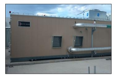
• Forced air cooling via raised floor data center fed by five (5) 500-ton cooling towers and dual-fed high efficiency computer room air handling (CRAH) units (left).
